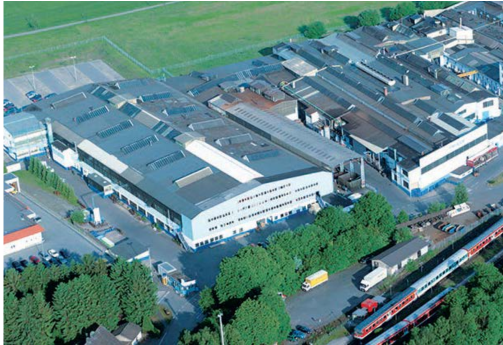
Bird's-eye view of the Thiele Schmiedetechnik plant in Iserlohn-Kalthof/Germany.
